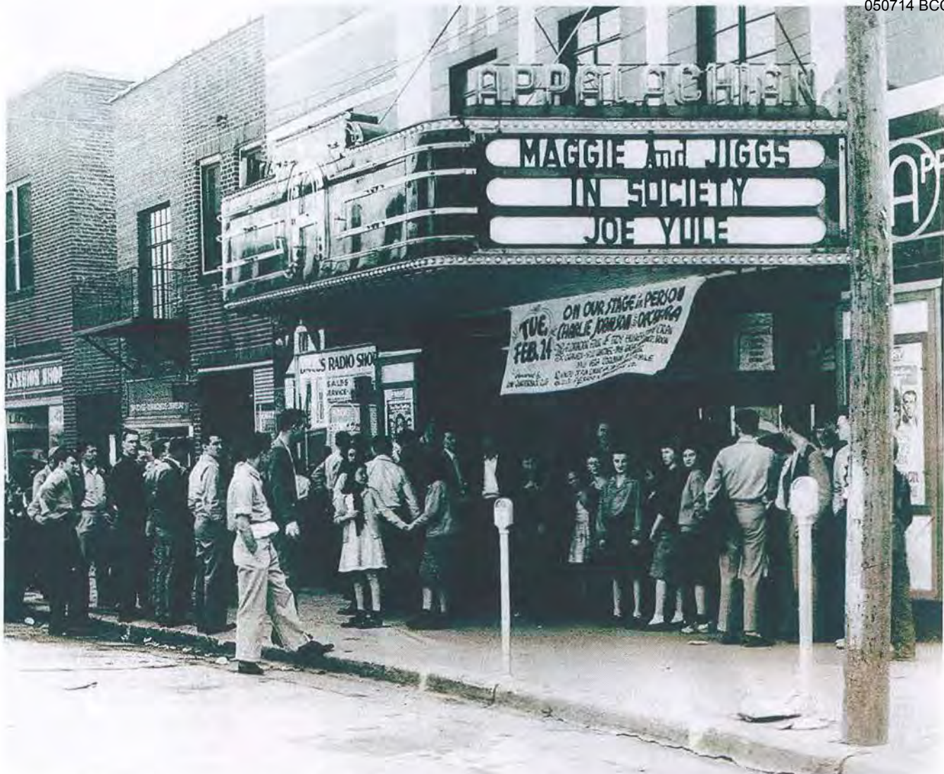
The projecting marquee (top) was neon and the original, exquisite front façade featured decorative, black-baked porcelain tiles arranged geometrically, leading to a prominent motif above the marquee. (see opposite page)
