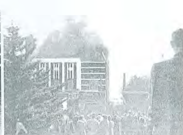
An unidentified man on the porch of the Daniel Boone Hotel (demolished in 1983) watches the devastating fire at Appalachian Theatre on Jan. 21, 1950, while escaping movie patrons gathers on the sidewalk. Photo courtesy of Watauga Democrat.
